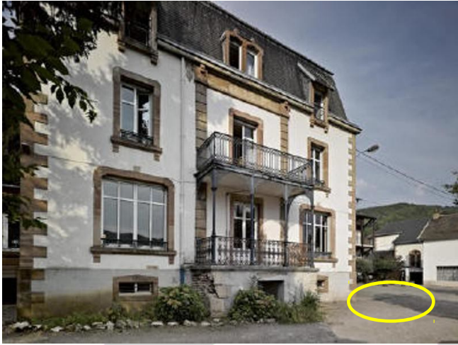
Bâtiment principal / Main building
